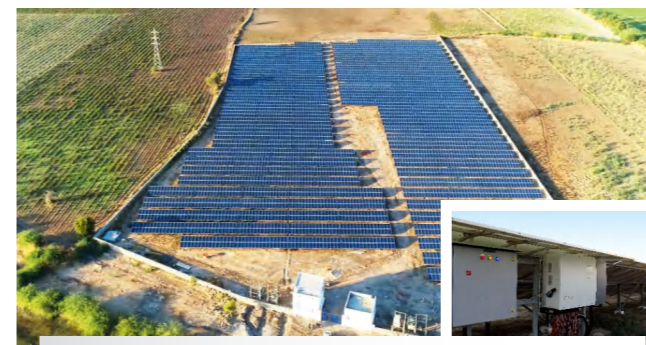
📍 Indie ⚡ 2MW 📦 Solis-(100-110)K
